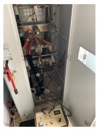
Fig .7. Connection of audio frequency generator to AABI-10 3x95 cable
